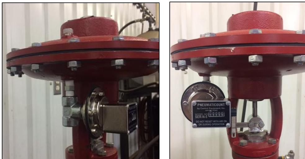
Figure 4-2. Model SERN-5 pneumatic counter (not fully installed)
