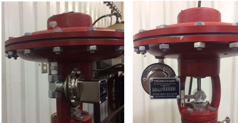
Figure 1. Model SERN-5 pneumatic counter (not fully installed)
