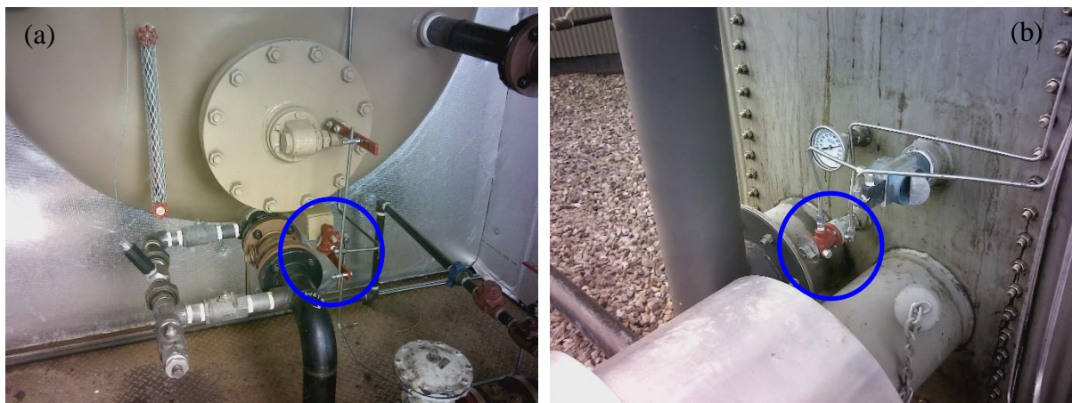
Figure 3-2. Examples of well pad PCs: (a) separator PC and (b) thermostat PC on tank
